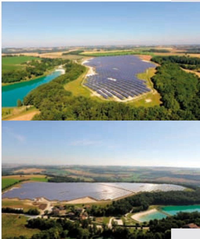
▲ «Saint-Clar» Project : Our 9 MWp Solar Park
